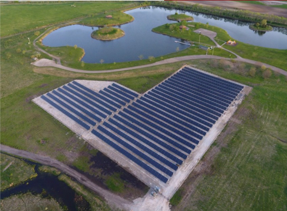
(Pictured below) Rantoul solar site
